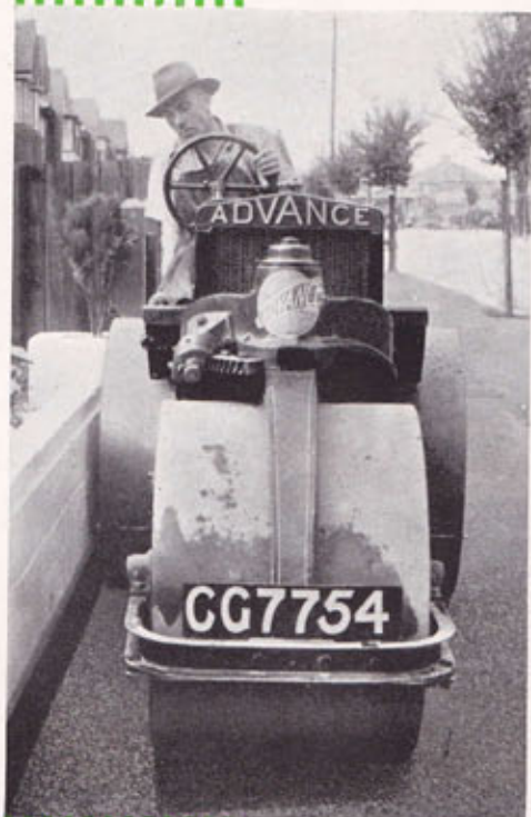
ABOVE (ON LEFT), BOTH SIDES CLEAR. YOU CAN ROLL CLOSE UP TO EDGE OF WORK. (ON RIGHT), A WIDE RIM MODEL.
