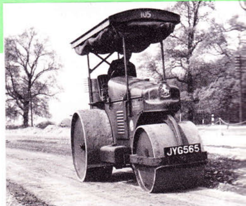
On a road re-location job, this type 'GBV' Roller is consolidating the sub-base.
