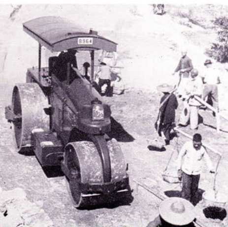
Hong Kong. A 'GD' consolidates a fill in the course of re-routing the Island Road at Shaukiwan Hill.
