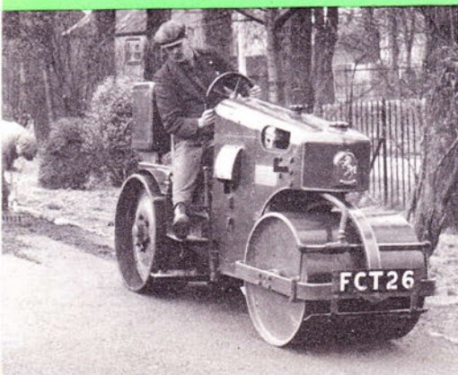
This 'GA' Roller is seen rolling the pathway through a municipal park in England.
