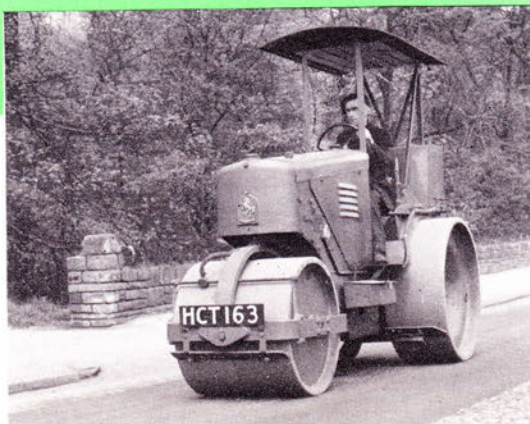
A type 'GF' Roller surface finishing a road near Sheffield.
