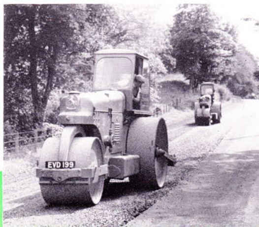
Two type 'GD' Rollers re-surfacing a road in Lanarkshire, Scotland.
